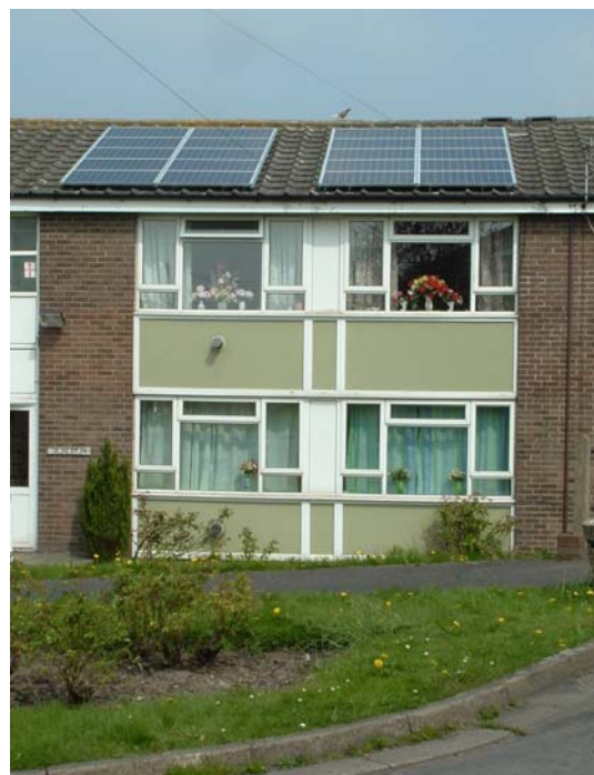
Solar PV panels installed at Primrose Hill
