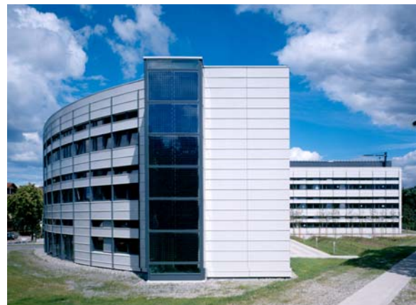
Figure 5: View on the facade of the access tract (photo: Guido Kirsch)
