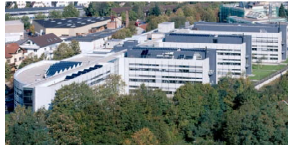
Figure 1: The new premises seen from south-east, before mounting of the PV system at the spandrel of the south facade (photo: Guido Kirsch).
