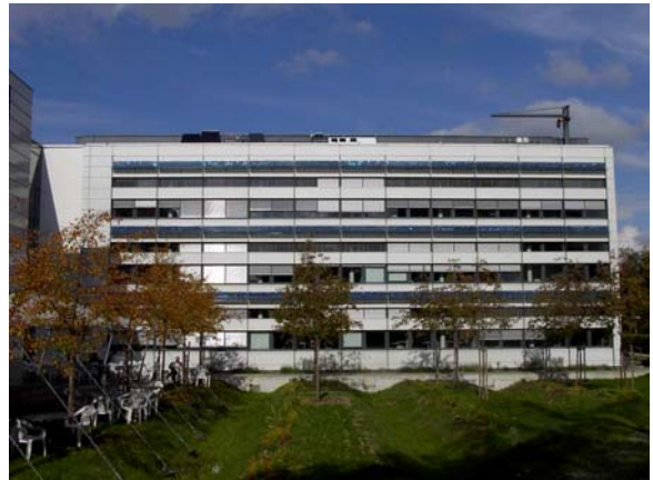
Figure 14: A view on the facade of the south wing
