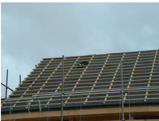
Counter battens (verticals) installed correctly for cooling, beneath battens
