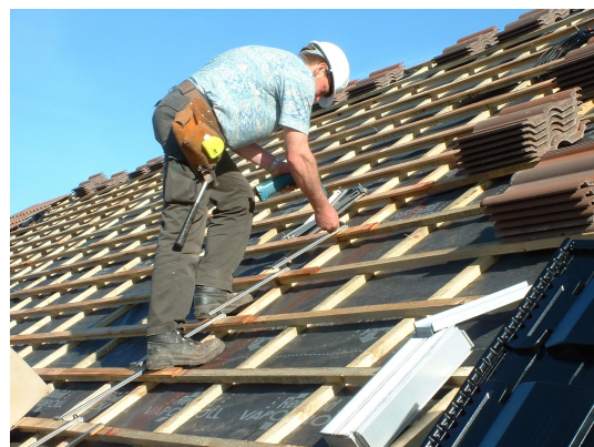
Mounting brackets being installed
