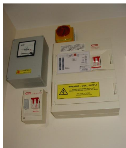
Tenant display meter (top left) mounted next to the consumer unit
