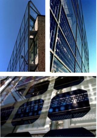
Figure 1. Photos of the facade with PV cells.
